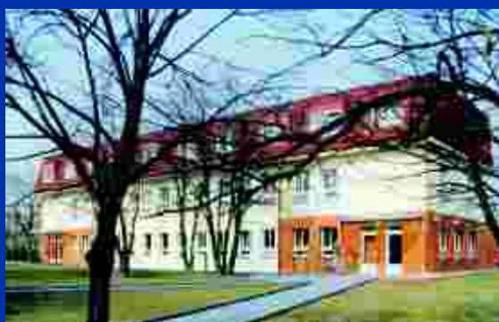
Centrum Paraple, Praha 10
